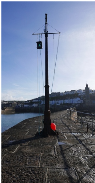
The mast on the Pier
