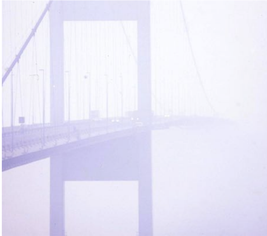
Figure 2. Severn Bridge in fog, c. 1979.
