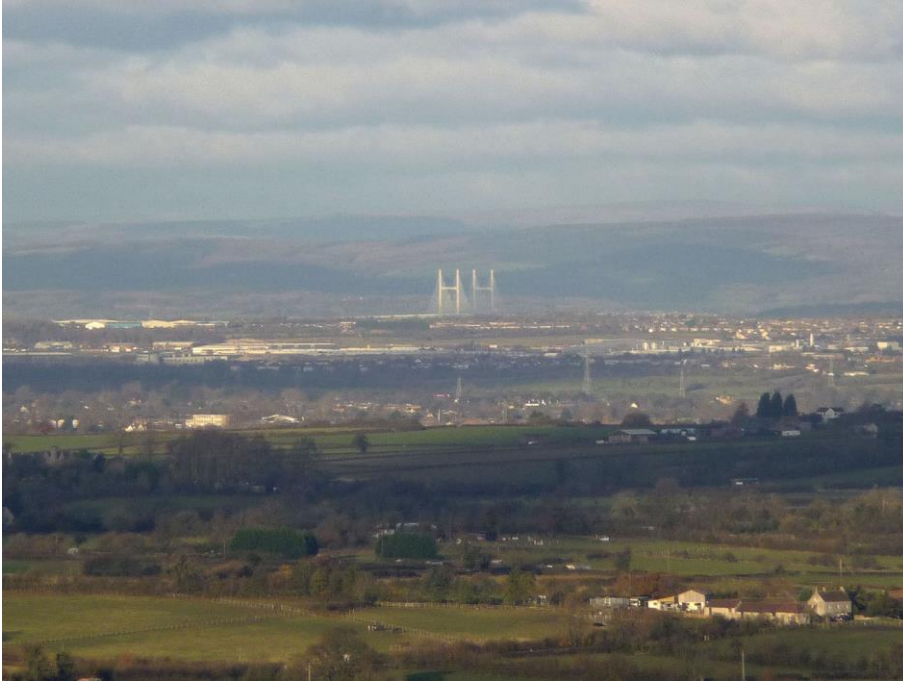
Figure 1. Second Severn Crossing, 2010. England in foreground, Wales in left distance (all images by author).
