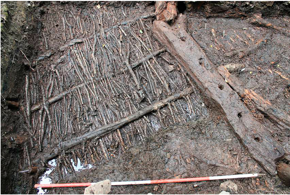
Figure 5. Sillbeam 223/1 in situ displaying stake holes and jointing around the posts. The stakes of the outer wall are visible to the left. The wickerwork screens formed the sub-floor of the Phase 1 building.
