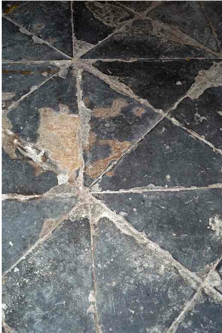
Fig. 24 Chipped and water damaged flooring in the crypt
